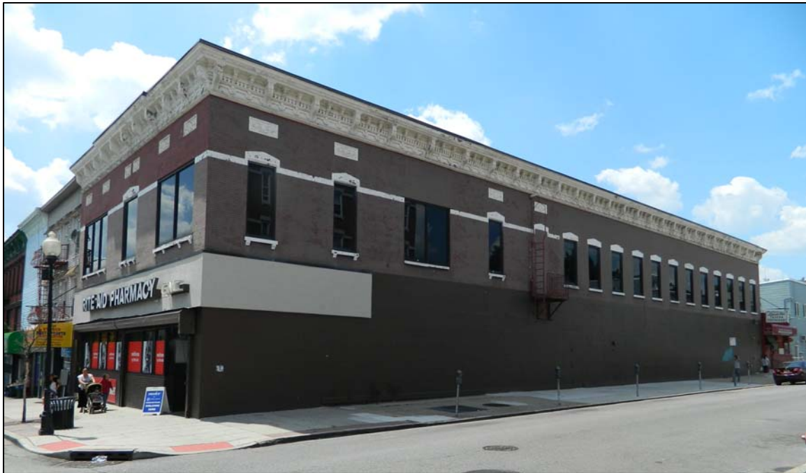
Wall space at 337 Central Avenue, Jersey City NJ
