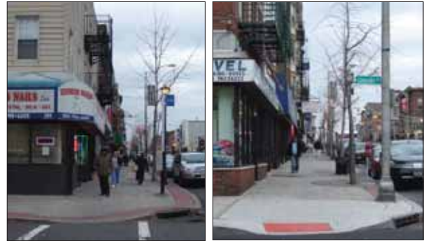
The corners of Central & Griffith and Central & Lincoln, showing the traditional curb design and the new ADA-compliant design.
